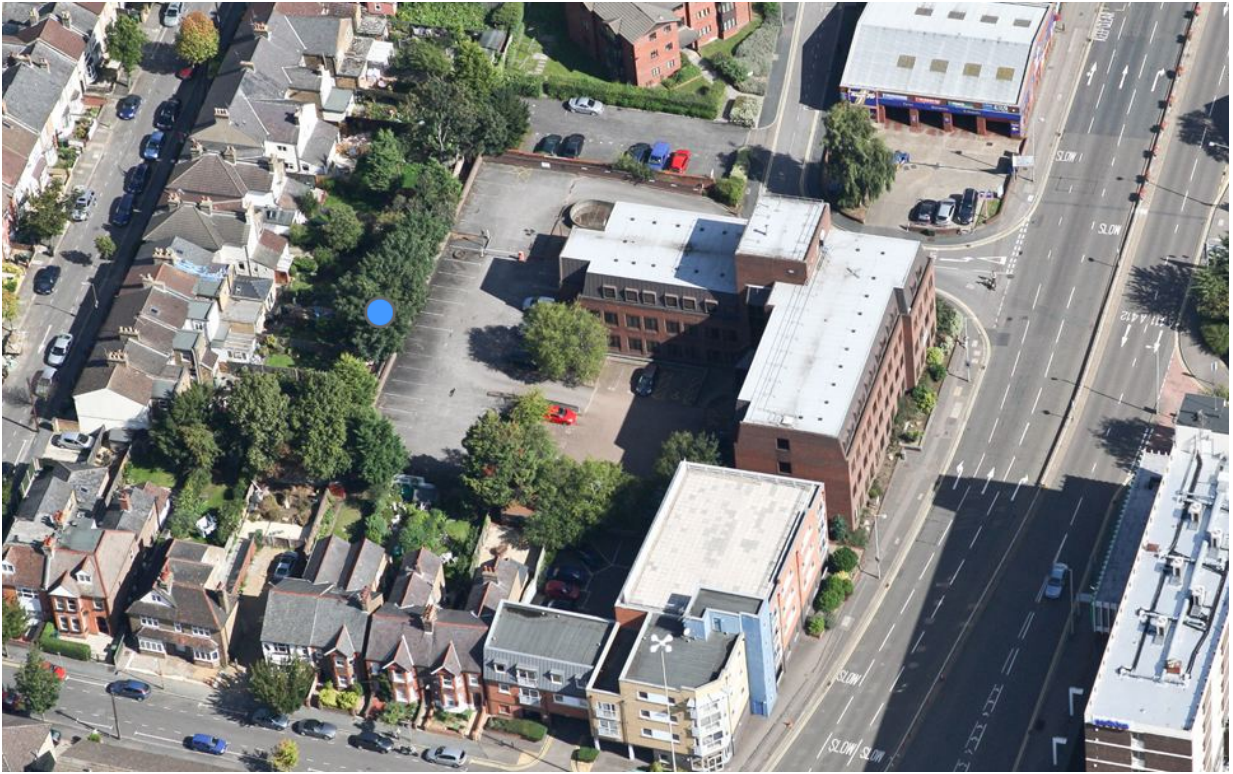
Fig.1. Aerial view of site.
